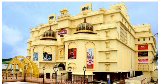
Capital Mall Udaipur – 10 Units
